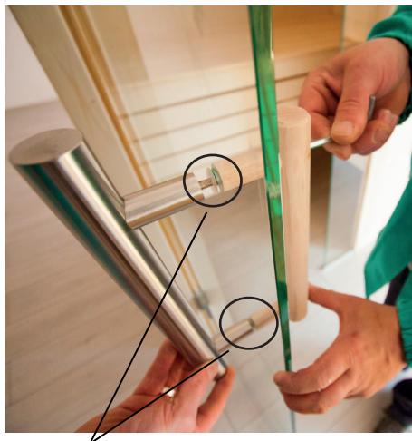
Attach plastic washers on the stainless steel handle
